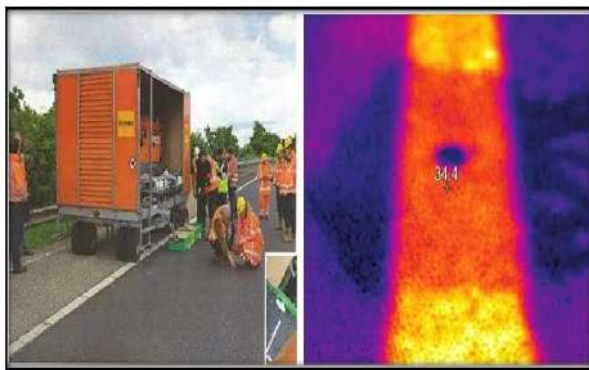
Fig. 3.: Induction heating in-situ
